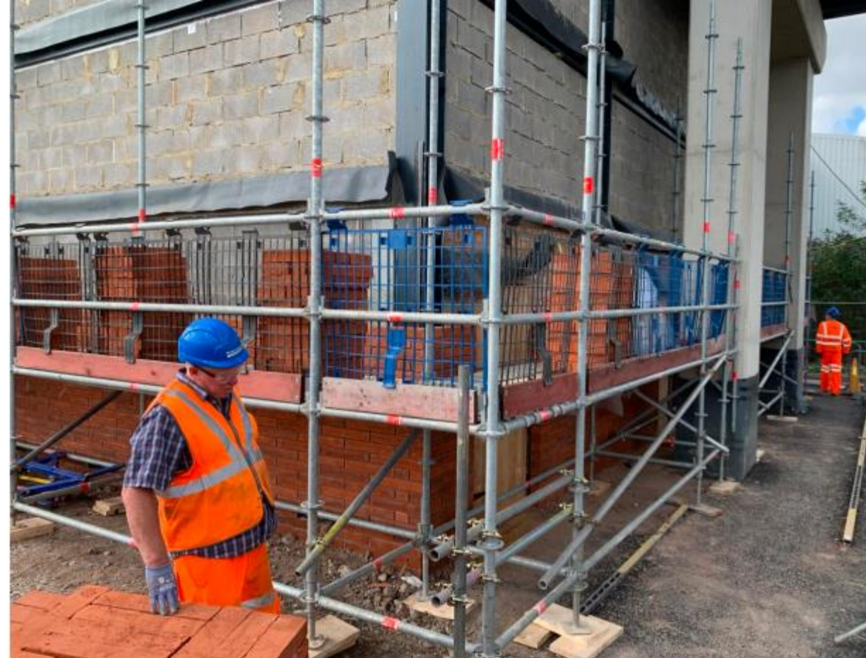
WEB brickwork onto the second lift
