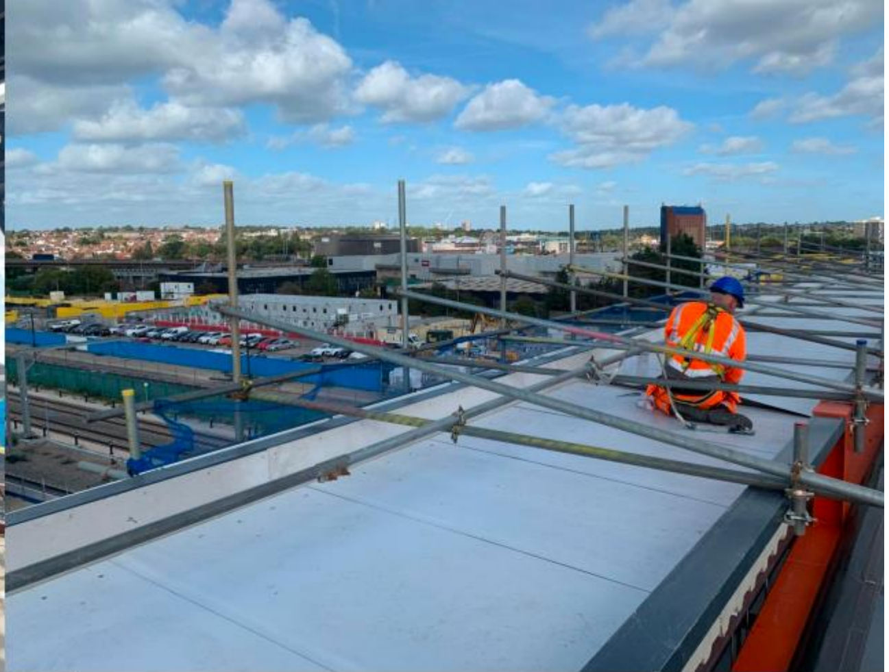
GL:1 roofing completed
