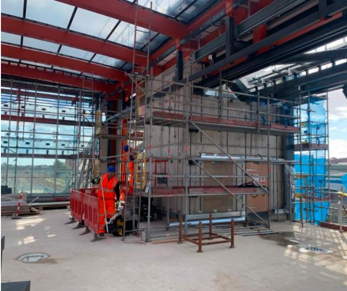
FourWays installing conduit to Fast platform lift shaft
