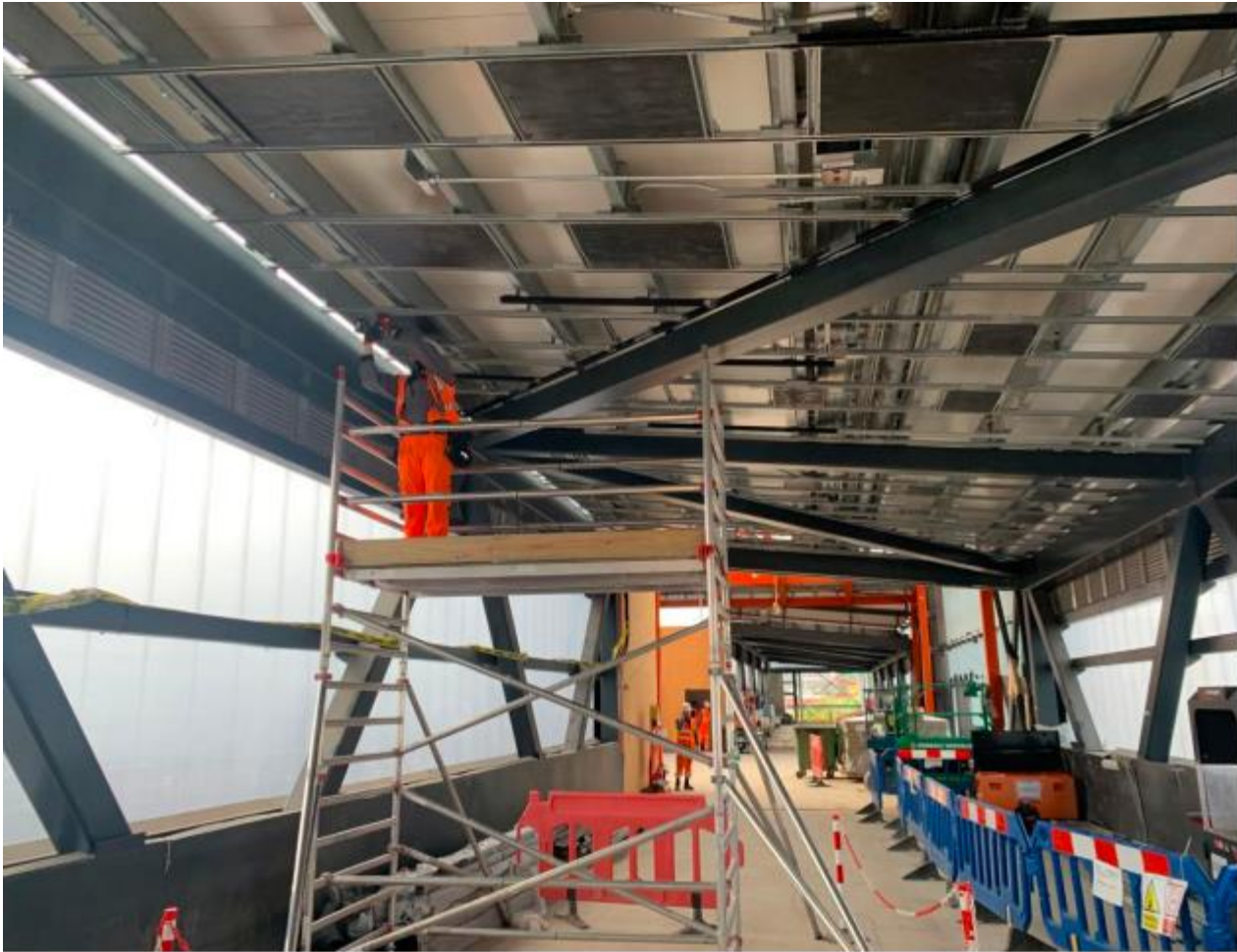
Lindner installing ceiling grid
