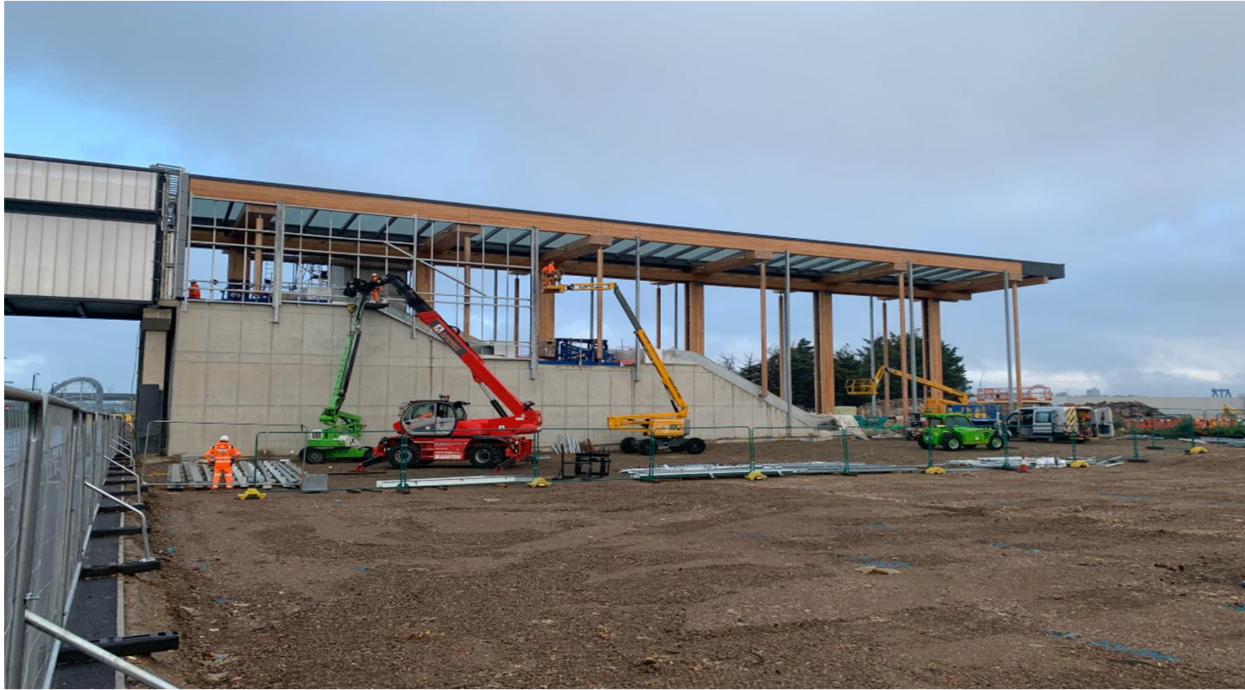
SEEB – South Elevation Hoarding
