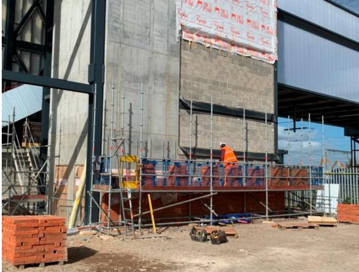
WEB brickwork onto the second lift
