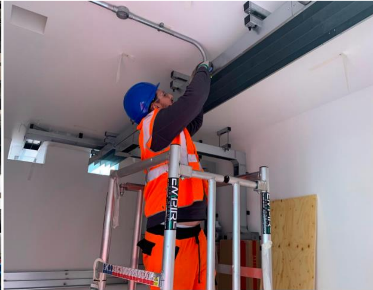
Fourways installing CMS to the LV switch room
