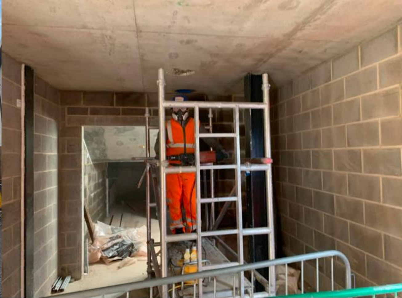
WEB BWIC holes to walls and slabs in progress
