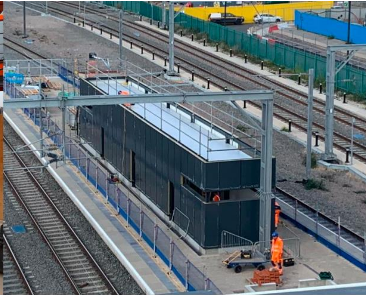
Drivers accommodation roofing installed
